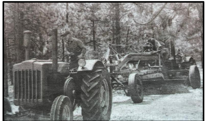
Dwight, Andrew, and Joel Zeller grade a new road through the seminary campus. Circa 1975.
